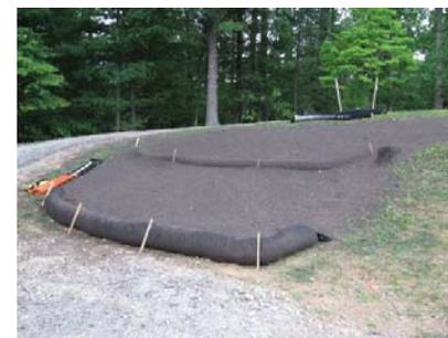
*Compost mulch used as a ground cover and as a fill in a check dam.*
