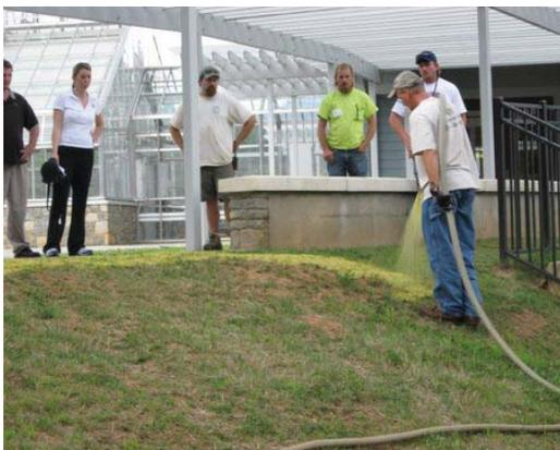
*Hydraulically applied mulch used for erosion control.*
