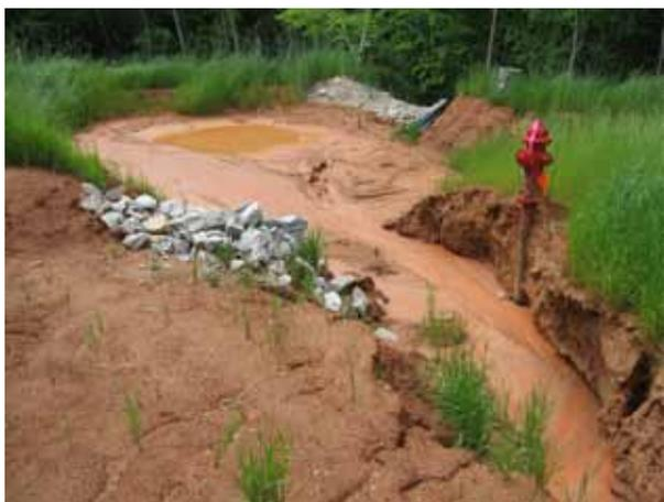
*Fig. 2 First place. Massive erosion exposing main water pipe to fire hydrant.*
