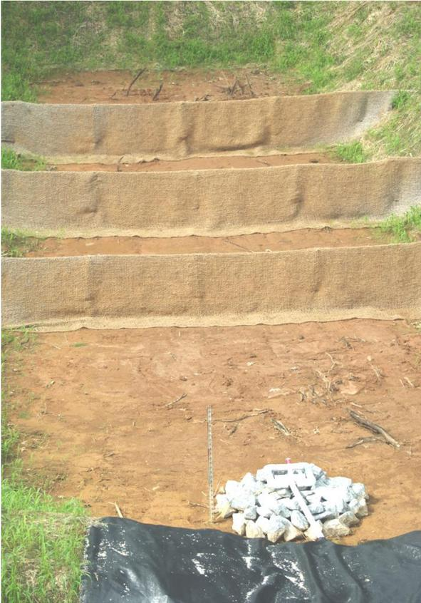
**Figure 6.65c** Example of porous baffles made of 700 g/m<sup>2</sup> coir erosion blanket as viewed from the outlet.
