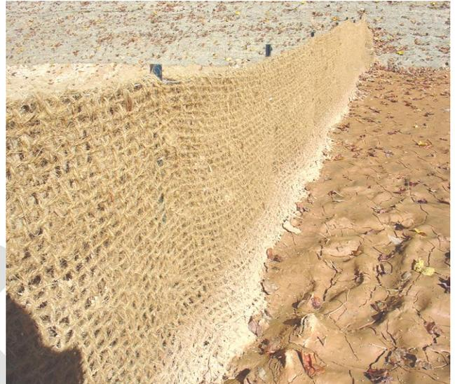
**Figure 6.65d** Close-up of a porous baffle.
