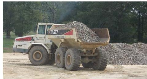
**Crushed screened concrete is transported to a staging area to be sold or used as road-base on site.**
