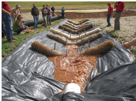
Figure 1. Wattles installed with PAM.
