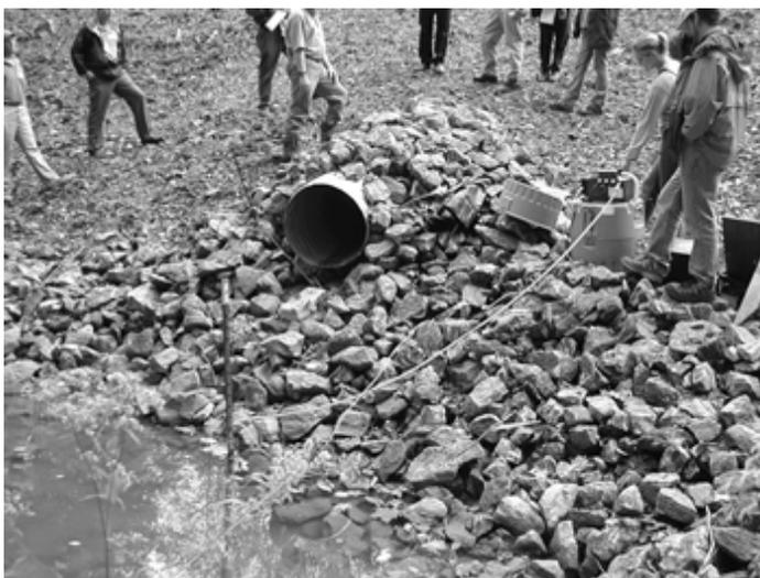
A PAM floc log is secured just below the basin outlet pipe where flow will dissolve more PAM and encourage flocculation in this settling pool, which is at the end of the PAM-BMP train. Sampling here has shown turbidity as low as 50 NTU.
