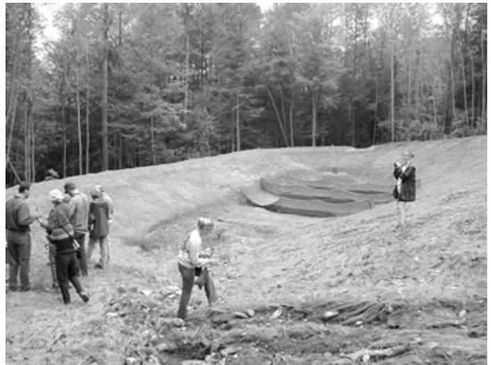
Jute baffles in this large riser-barrel basin have slowed water velocity and encouraged sediment to drop out in forebays just below the inlet. One side of the first baffle has collapsed. McLaughlin recommends using tree protection fence as the first baffle because it can better withstand the force of water rushing into the basin.
