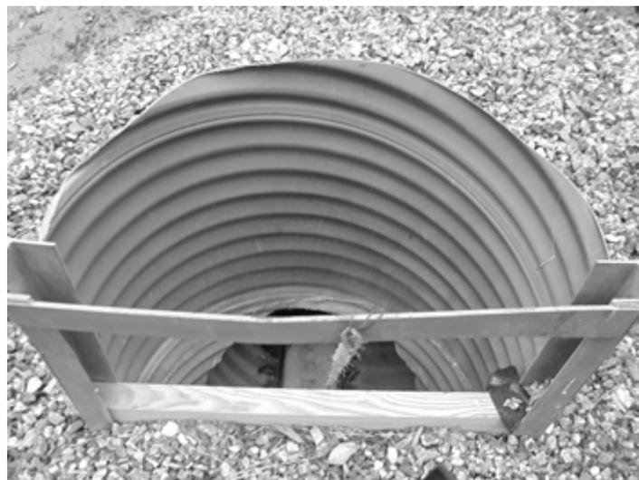
The traditional riser barrel has been replaced with a flashboard riser that allows the researchers to retain water in the riser and pool. A PAM floc log is suspended in the barrel. McLaughlin says this is the ideal place to use a floc log.
