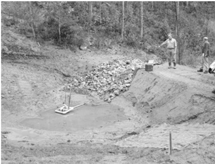
A skimmer improves the effectiveness of this sediment trap in removing sediment from runoff. Sediment must be removed from runoff before treating with PAM to reduce turbidity. Dr. Rich McLaughlin points out erosion at an inlet on the far side of the trap. "Inlets should be protected," says McLaughlin, "otherwise, the trap fills up with sediment eroded from its own banks. That's silly!"
