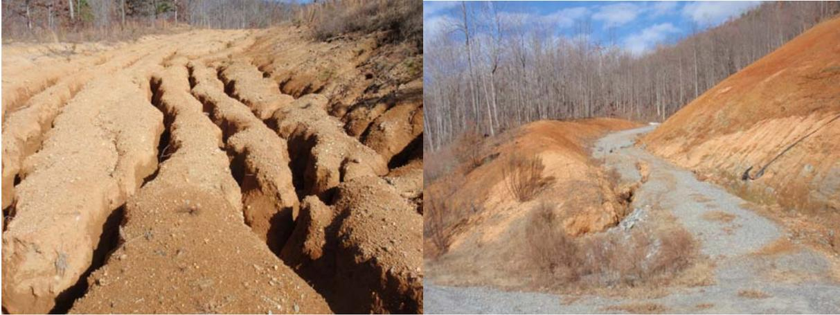
*Examples of abandoned construction sites with eroding roadways and slopes causing offsite sedimentation.*
