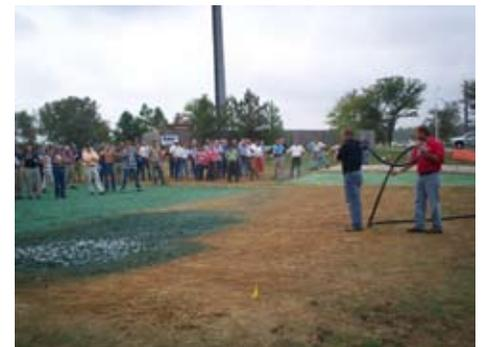
*A demonstration of hydroseeding as an application of mulch used for ground cover.*
