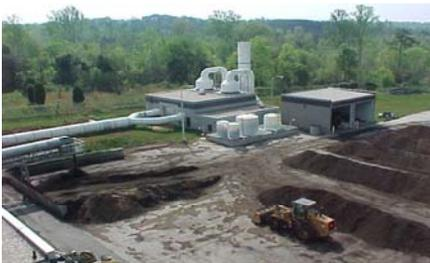
manufacturer. It is stored in a 26,500 cu. ft. silo and the facility recently upgraded and installed a centrifugal separator and kept the two old belt presses as backup. After separating out the solids (approx. 9.8 tons per day) at 3.5 percent solids, the sludge/sawdust mixture is then fed into one of four reactors. Each reactor is 63' long, 18' wide and 12' high (13,608 cu ft) with a capacity of 20 tons per day. The system is designed to provide a 14
