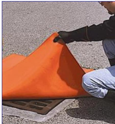
When vehicle washing is performed in the vicinity of a storm drainage collection system, cover the storm drain with a portable drain cover to prevent illegal discharges.
